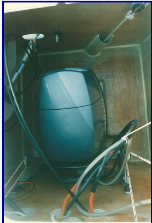
Outboard installation aft of cockpit bulkhead.
