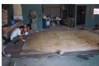
Cabin roof is strip-planked.
