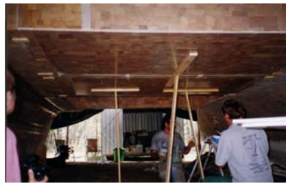
Bridge-deck goes up
