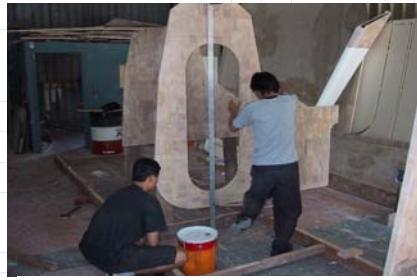
Standing the bulkheads
