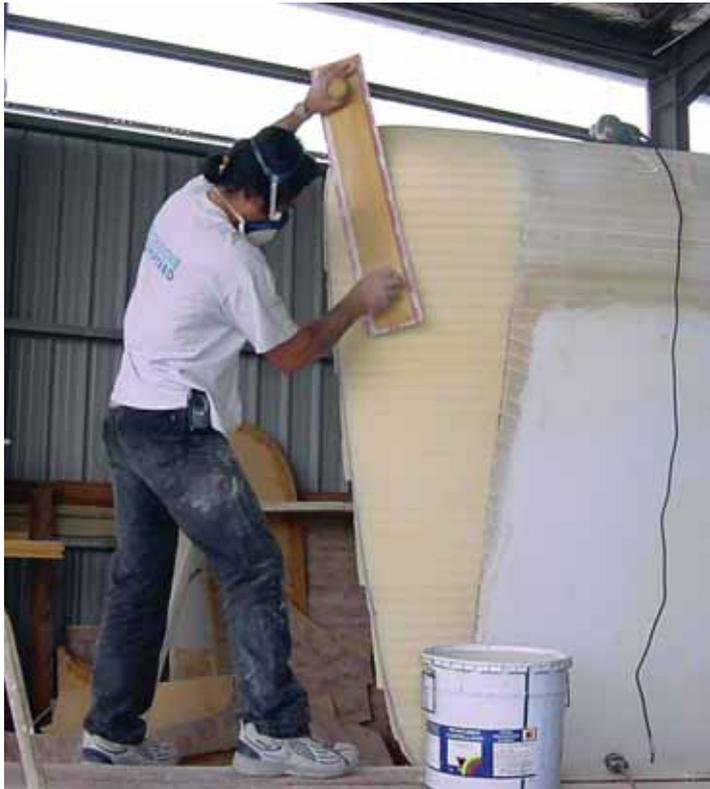
4. Once the tops of the ridges have been sanded, fair with 80 grit sand paper and a long sanding block. Use a straight-edged squeegee to trowel a second application of fairing compound over the surface, filling the grooves. The compound should be flush with the ridges, leaving only minor sanding before finishing.
