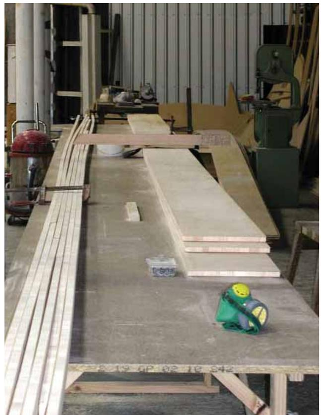
Building a plywood table at a comfortable height for working is a great back saver when compared to working off the floor. The table must be the length of the longest strip being constructed. That is, if you are gluing five 2400mm DuraKore strips together to form a strip 12 metres long, your table must also be 12 metres long.
